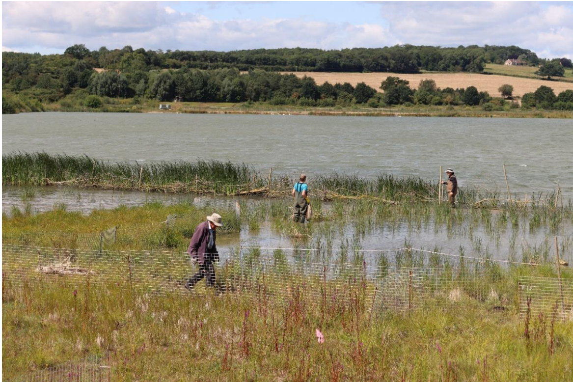
A belt of Lesser Reedmace forms the outer perimeter of the northern part of Flasks Fen, reinforcing the dead hedge as a wave-break and silt trap. Planting in sandbags is safer and easier for our volunteers.
